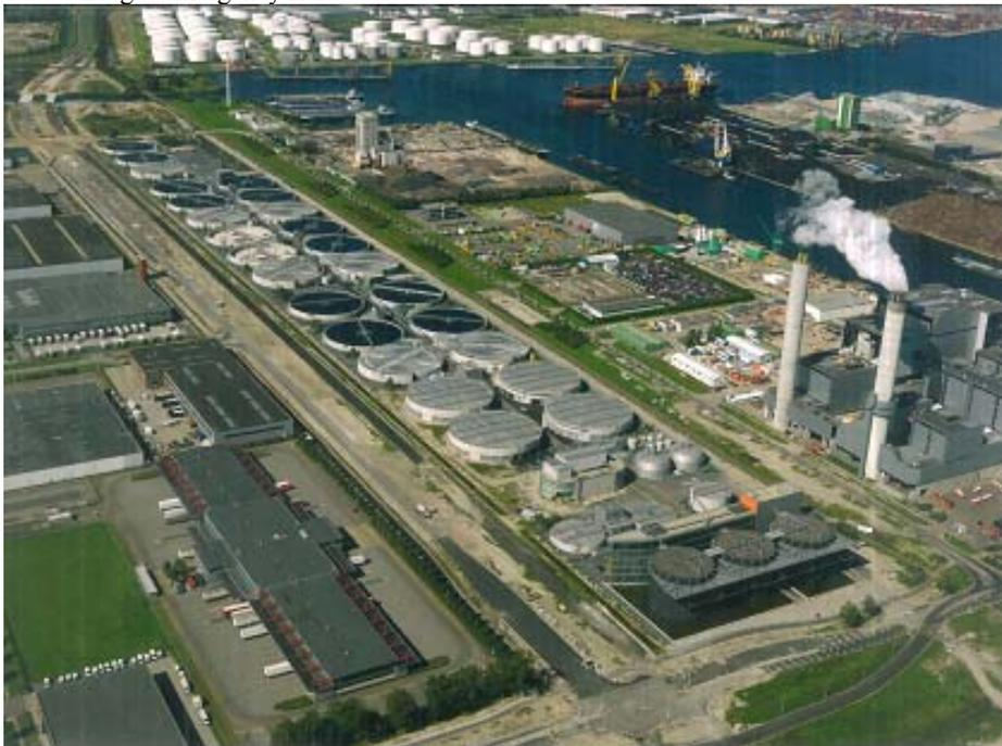
**Figure 1.4** Aerial picture of the WWTP Amsterdam West. In front: digestion tanks with office buildings and sludge treatment, in the background: the wastewater treatment lines, and on the right side: the AEB.
